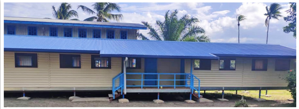
St Joseph Technical College, front view of the double classroom at the St Joseph Technical College. Each classroom can accommodate 40 Students.
